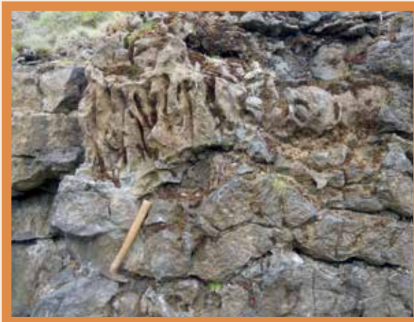
At the west end of the quarry the rock becomes brown in colour, which may be due to alteration of the limestone from faulting and the proximity of the igneous sill.
